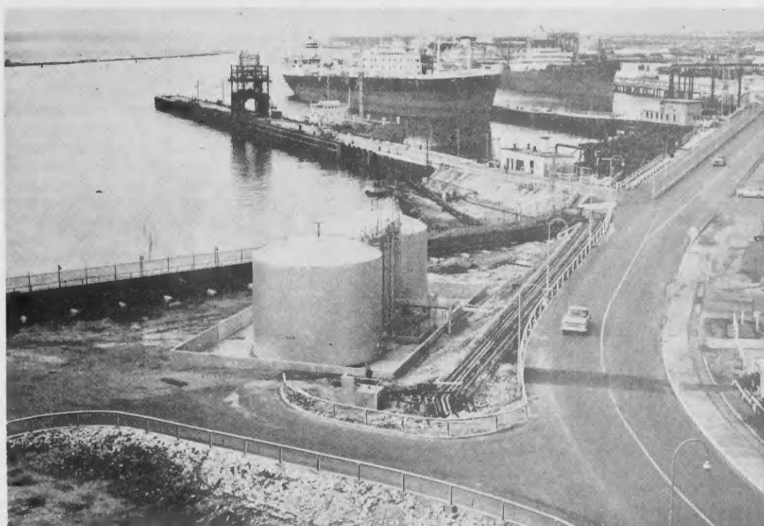
THE NEW tetraethyl lead system of storage tanks and lines is unique at Lago. Ethyl Corporation owns the compound until it reaches weigh tanks in the blending plant.
